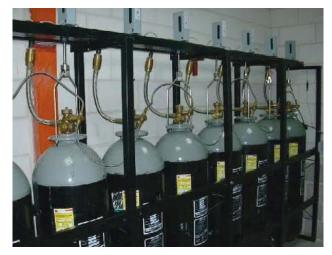
CO<sub>2</sub> extinguishing system in paint booth
