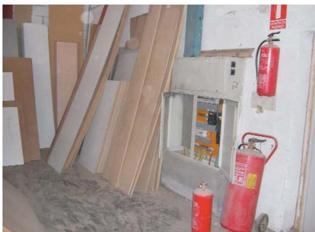
Pile of wood close to switchboard
