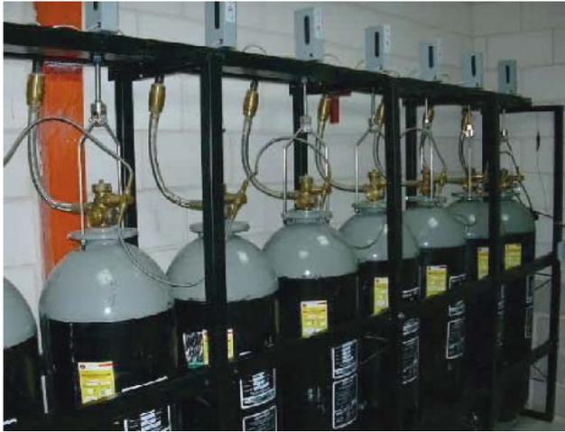
CO<sub>2</sub> extinguishing system in paint booth
